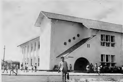
One of Oranjestad's most beautiful new buildings is this recent addition to the Juliana School. Un di e edificionan di mas bonita na Oranjestad ta e school nobo aki cu ta un parti di Juliana School.
